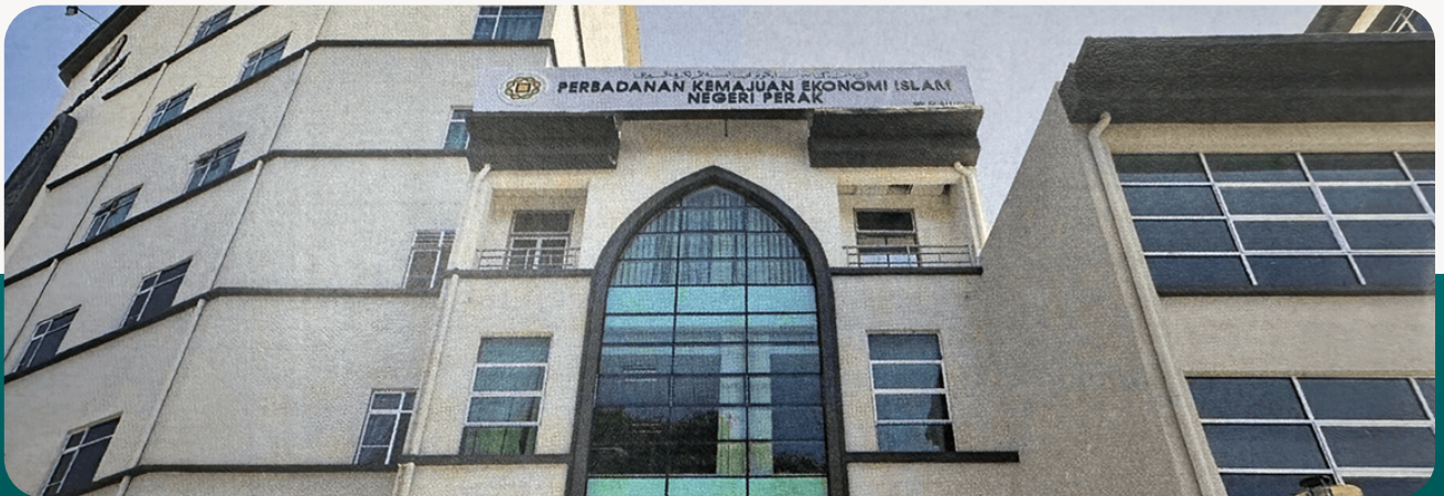
PSB Office Building, Greentown Suria
