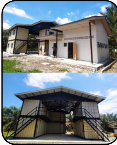
Worker Quarters (Container & IBS type), Gelung Pepuyu Estates
