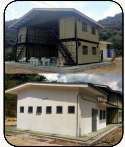
Worker Quarters (Container & IBS type), Sg. Charok Estates
